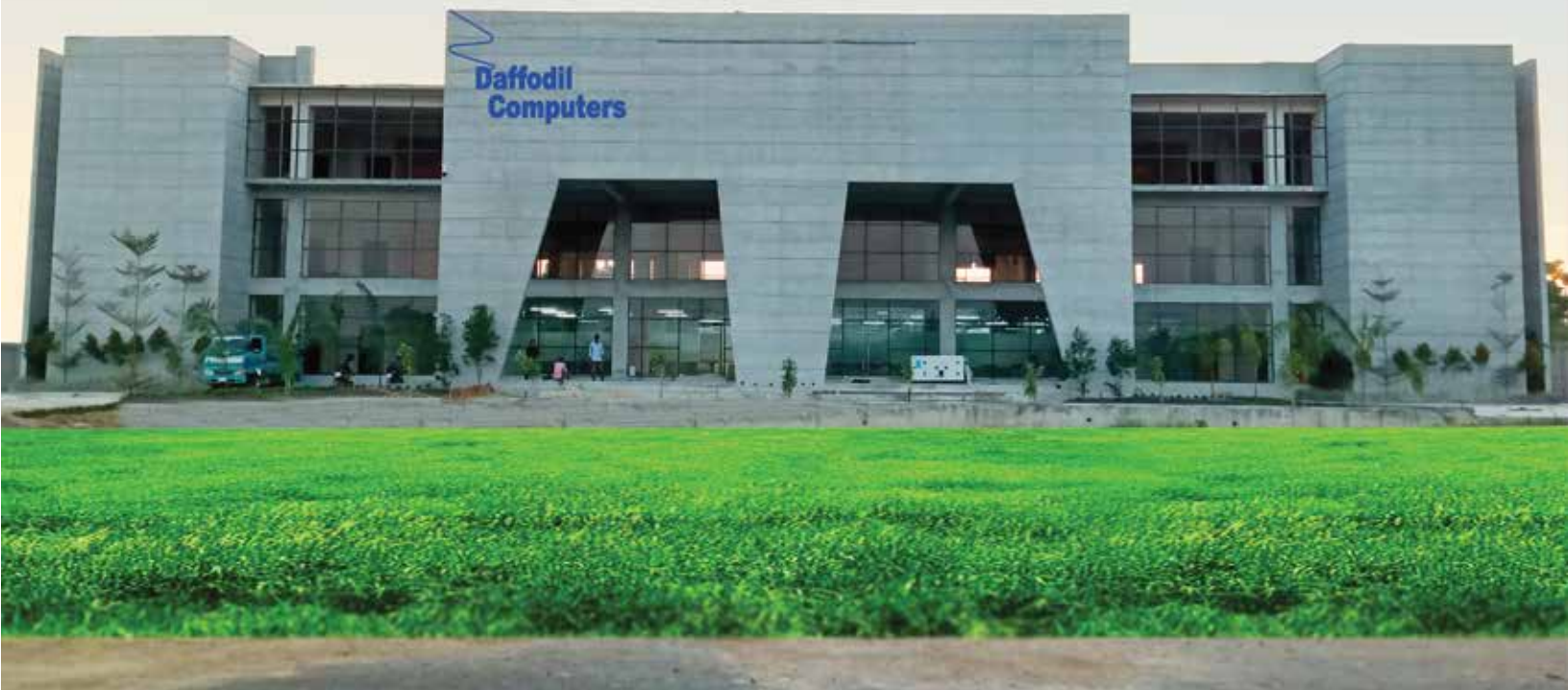
P.S.: PRESENT BUILDING PHOTO OF DAFFODIL COMPUTERS LTD. ASSEMBLING AND MANUFACTURING UNIT, BANGABANDHU HI-TECH CITY, KALIAKOIR, GAZIPUR
